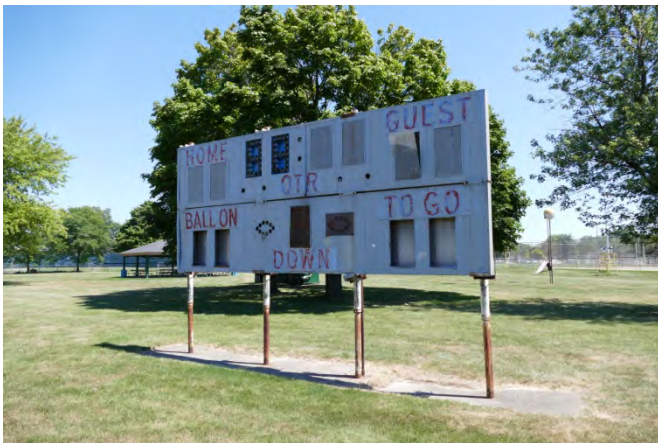
Dilapidated score board
