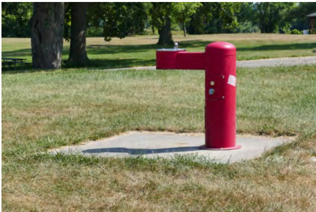
Existing drinking fountain
