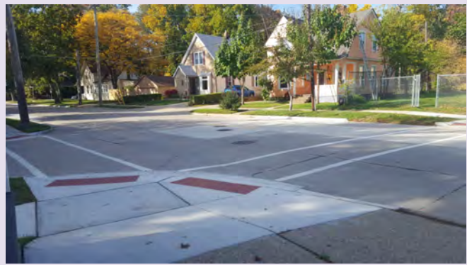
Rebuilt sidewalk ramp on Church St.
