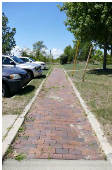
Brick paved path
